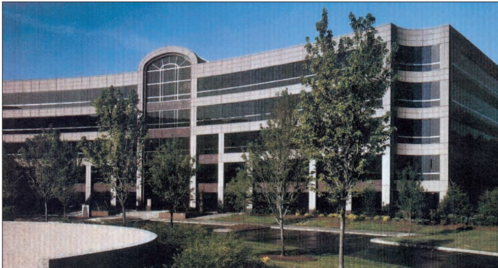
The new location of the Executive offices of The Academy of Medicine of Cleveland & Northern Ohio in the Park Center Plaza on Rockside Road.
